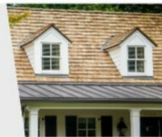
Wood Shake Roofing
