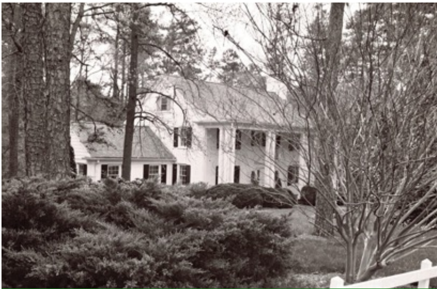
Braibanti House, 3805 Darby Road (1954)
