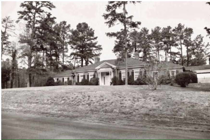
Sloan House, 3232 Westover Road (1961)
