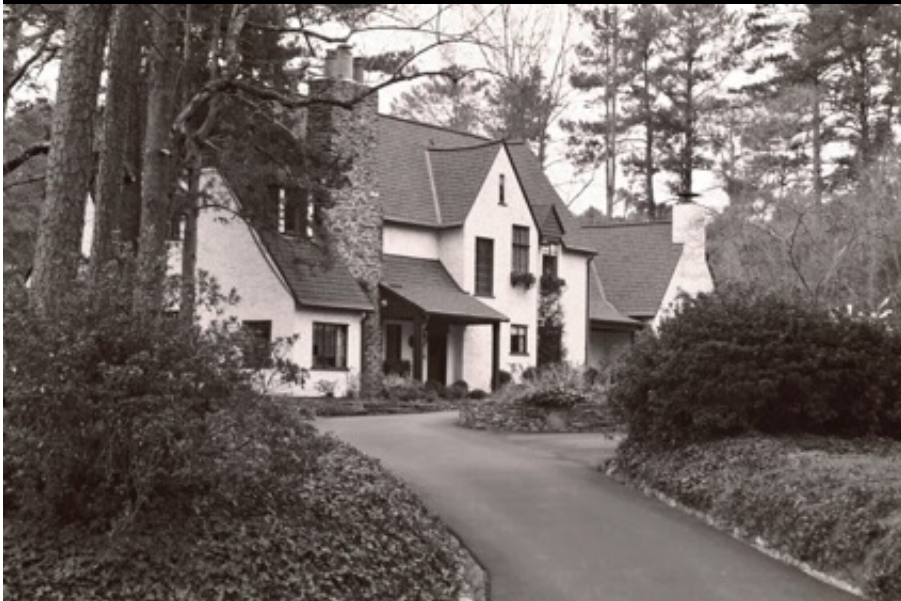
Snow House, 3301 Devon Road (1928)
