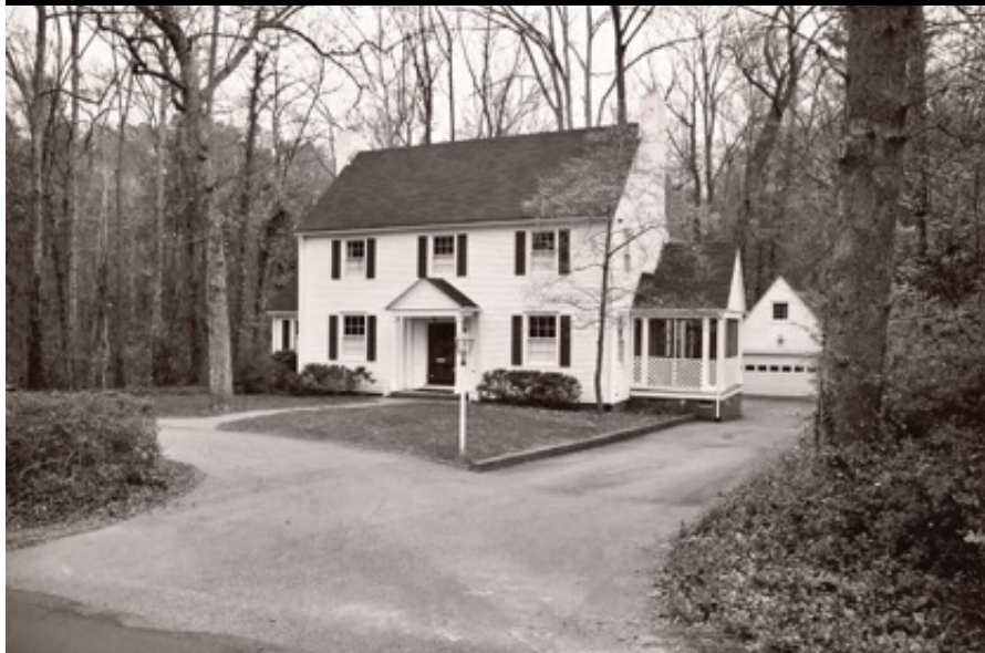
Eadie House, 3433 Dover Road (1930)
