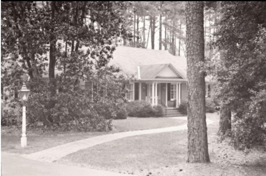
Montgomery House, 3407 Windsor Way (1956)
