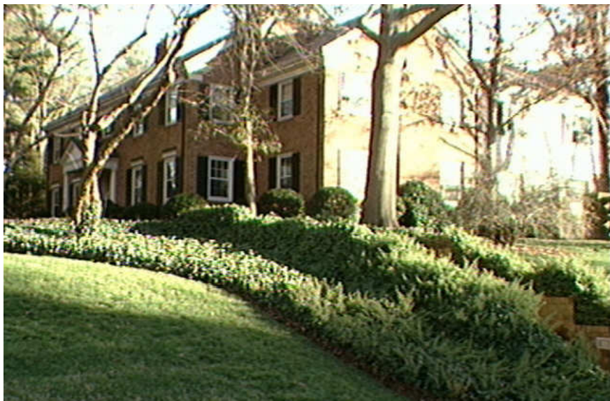
Harris-Teer House, 3900 Dover Road (1956)
